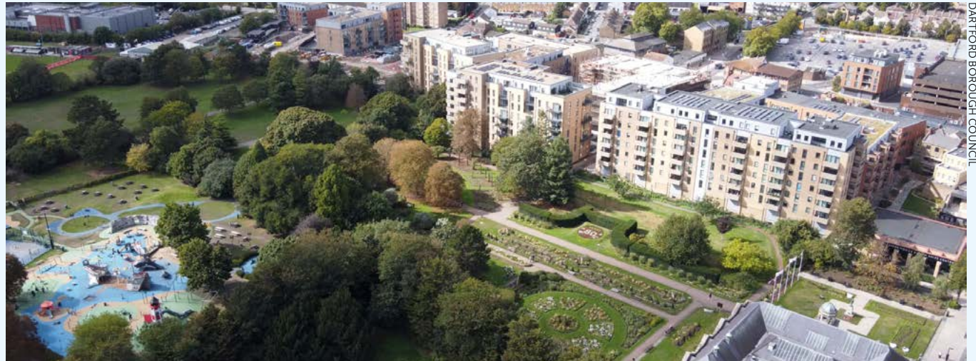
Bellway Development, Lowfield Street, Dartford.
