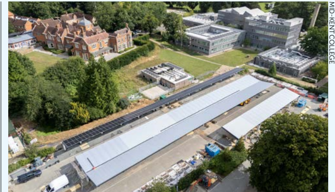
Solar carports at Mid-Kent College.
