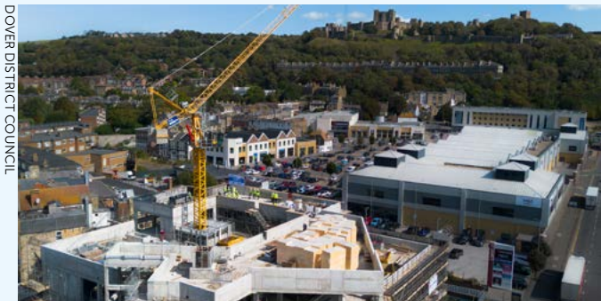
Construction of The Bench, Dover.
