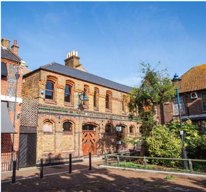
Old Wine Warehouse, 1 Charlotte Court.
