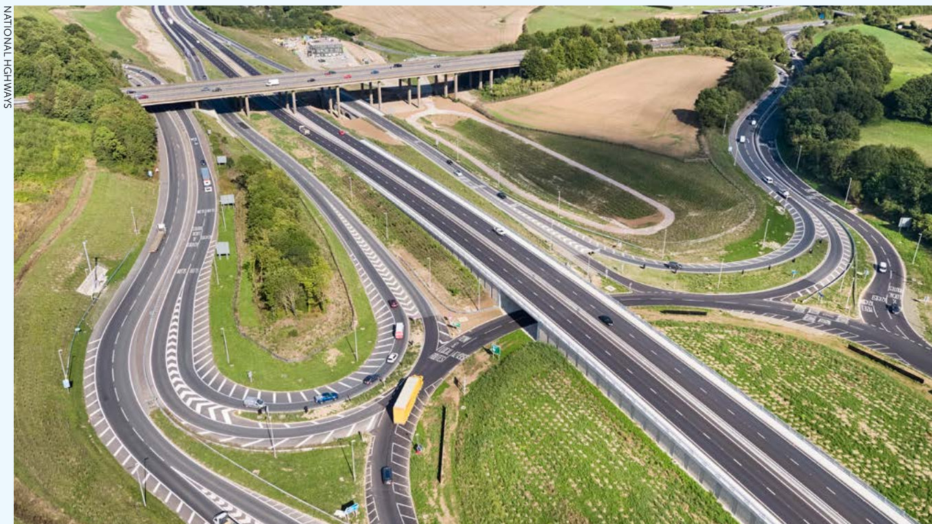
Completed works at Junction 5, M2.
