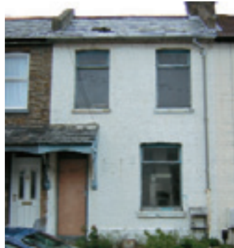
WINCHELSEA TERRACE, DOVER - BEFORE
