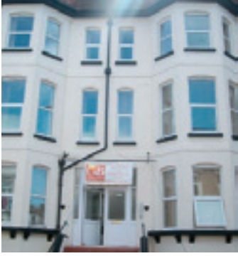
14-16 ATHELSTAN ROAD, CLIFTONVILLE
