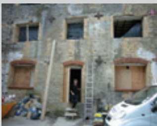
CAVES COURT - BEFORE
